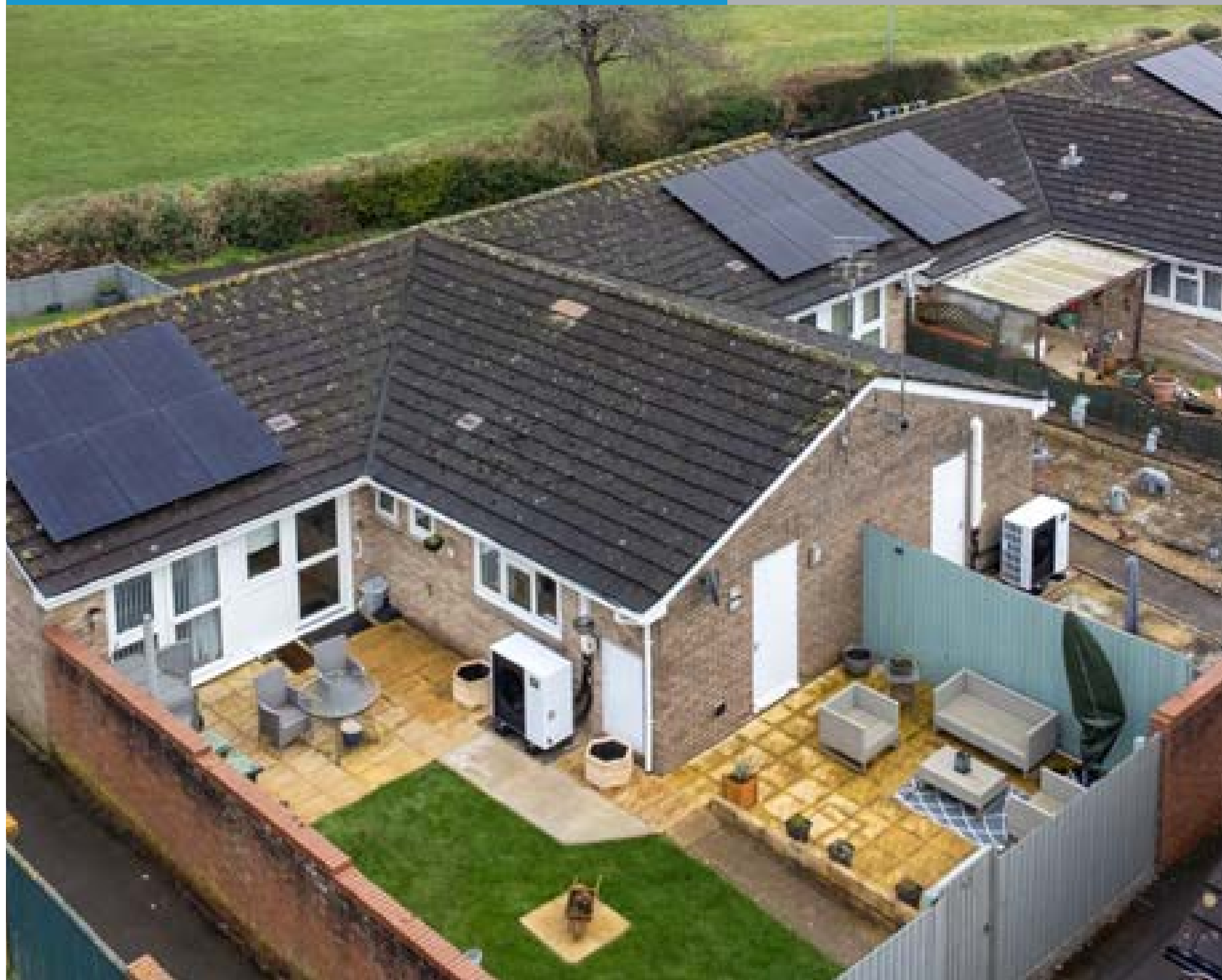
Some of our homes at Westcroft have received energy efficiency upgrades
